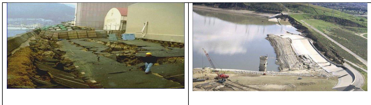
Fig-5.1 A- Soil Liquefaction
